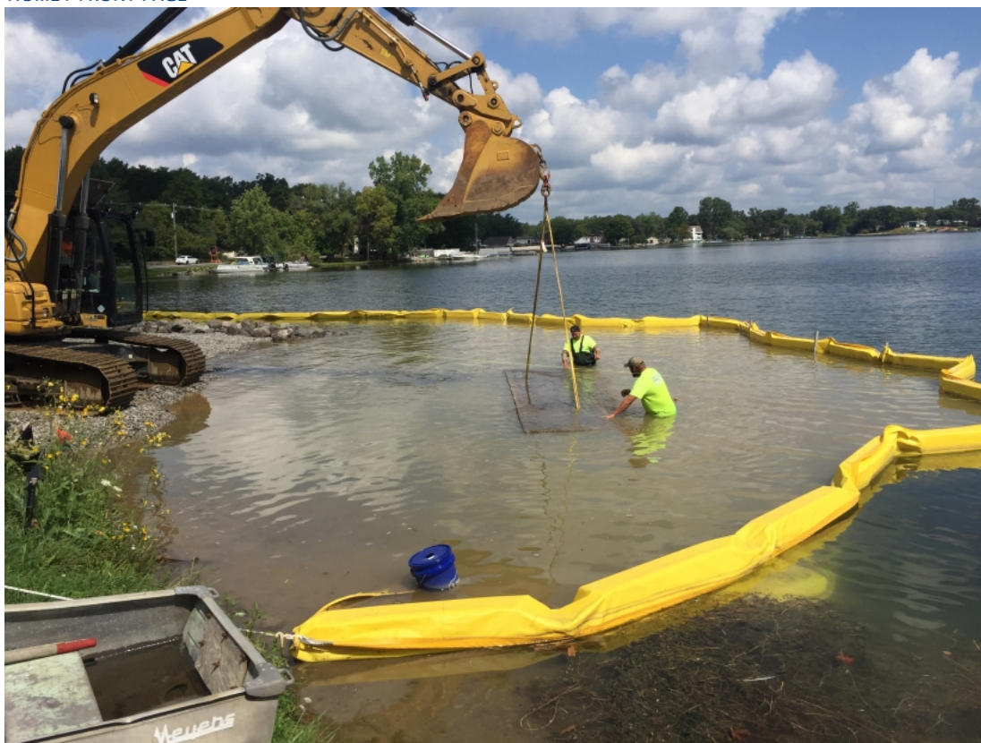
Construction crews work on the White Lake launch project.
